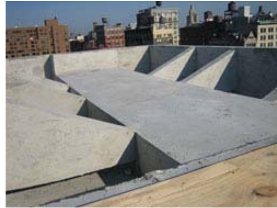
Figure 6 –Penthouse Roof Structure
